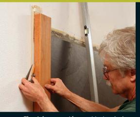
**The right setup.** After positioning the leg plumb side-to-side, shim it plumb to the wall. Set the compass points to the widest gap, then draw scribe lines down both sides of the leg.
