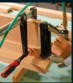
Add simple layers of trim. With the shelfand-frieze assembly turned upside down, dry-fit the two smaller layers of trim, then apply glue, clamp in place, and use a few pin nails to secure the miters.
