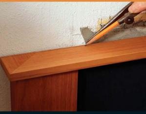
Adjust the reveal. To compensate for the uneven plaster, position the parting strip on the legs and use the compass to mark the amount to be scribed. The result should be an equal reveal over the legs on both sides.
