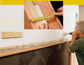
Attach the wall cleats temporarily. After measuring from the top of the shelf to the underside of the cleat (inset), transfer the cleat measurements to the wall. Use only one screw to attach each cleat so that it will be easy to adjust the cleat's position.
