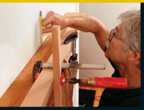
**Scribing with a crutch.** Instead of trying to hold the shelf in place while scribing, clamp a block to the shelf, then clamp to the block a long stick that reaches the floor.
