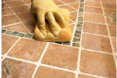
**Don't wait too long to wash.** The floor should be ready to wash after about 15 to 20 minutes; much longer than that, and the epoxy begins to harden. Make sure to wring out the sponge thoroughly before scrubbing. Too much water dilutes the epoxy, making it weak and discolored.
