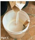
Mixing made easy. Combine Part A and Part B in a clean (preferably new) bucket, mixing with a margin trowel and rolling each bag like a tube of toothpaste to squeeze out as much liquid as possible. After stirring, add Part C, the cement-based colorant. Blend all three components until the mixture has a consistency similar to sticky cake batter.
