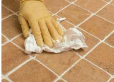
**Buff away the haze.** After both washes have been completed, use a cotton rag to wipe off the remaining haze. Avoid pushing down too hard with the rag; buff the surface firmly, as if you were waxing a car. Don't stop wiping the surface until every bit of sticky residue is removed. If you are working your way out of the room, make sure to watch out for footprints left on the tile surface.
