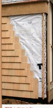
With a story pole tacked at each end of a long wall, nails partially driven into each course mark can be used to anchor successive chalklines. I tack a straightedge along the chalkline, arrange an armful of shingles across it, and nail them off. To keep loose shingles from blowing off on windy days, I sometimes stretch a taut string between the nails two courses above the one I'm working on.
