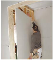
Hang it short. When a single panel will cover a wall or ceiling end to end between walls, cut it about ½ in. short so that it goes between the walls easily without binding on the framing.
