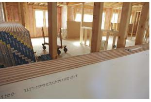
**Spread the load.** Spread the stacks of drywall out to avoid overloading the walls and floors. Then, when hanging, try to work off one pile until it's gone, freeing up the wall to be hung.
