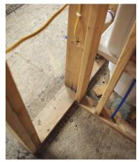
**Nailer needed.** You can safely float corners up to 8 in., but a short wall section like this requires a nailer.
