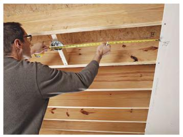
Screw it tight. Fasten panels along a long edge first, and then across the face to the other edge so the drywall pulls tight to the framing.
