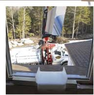
Check for fit. Before ordering drywall, ensure the panels will fit through doors or windows, and that those openings are accessible to a boom lift and are protected from damage. Here, a drywall slide is used over dunnage to protect the windowsill.
