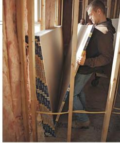
Bottoms in. When stacking drywall against a wall, the bottom edge of the first sheet should be 4 in. to 6 in. from the wall. For successive sheets, nudge the bottom edge into the previous, lower them to the floor, and lean them back to keep the stack tight.
