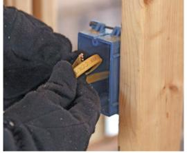
**Safety first.** Electrical cables need to be pushed into the back of boxes before the drywall is hung to avoid getting nicked by cutting tools.
