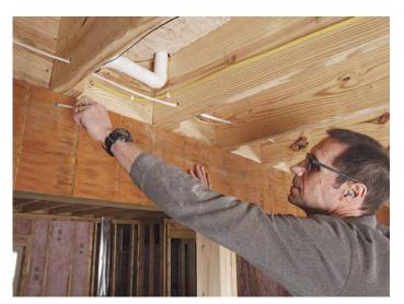
Mark for penetrations. For ceiling boxes, measure straight over from the edge of the wall or the previous panel to the center of the box, then write that measurement next to where you pulled it from so that it can be referenced and transferred to be cut out in place when the next panel is hung.
