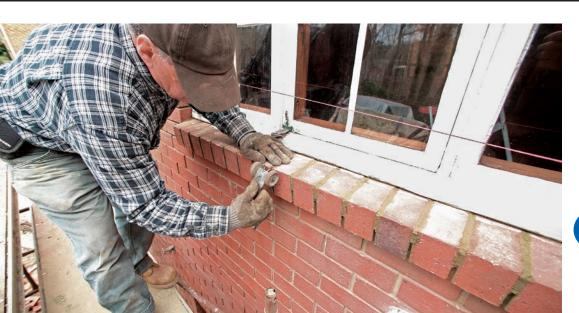
**The final raking.** To prevent blowing out the corners, rake the joints from the bottom halfway up, and then finish by raking down from above.
