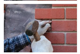
**Chisel where you must.** Use a 3-lb. hammer and a <sup>1</sup>/2-in. masonry chisel to clean up the remaining mortar. Tap lightly to avoid damaging the brick.
