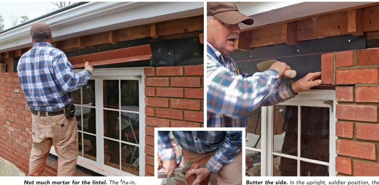
Not much mortar for the lintel. The 9/16-10. thickness of the lintel is close to that of an ideal mortar joint. To keep the courses consistent, only a little mortar was placed under the lintel.
