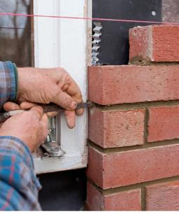
**Work in from the corner.** A joint raker won't fit where the brick returns to the window, so a tuck point is used instead. To make a crisp, mortar-packed angle, work the mortar away from the corner.
