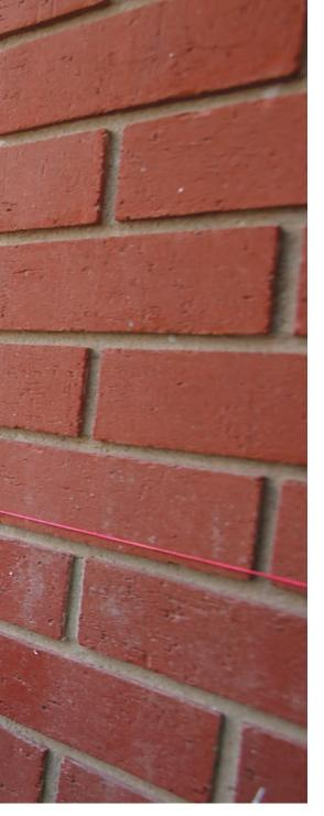
lighter and tanner in color than modern mortars, which are often gray. To match mortar, you'll need samples. Play around with different cements and dyes (*FHB* #258, pp. 60-65) and give your samples about three weeks to dry to ensure the closest match.
