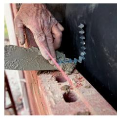
**Bed the wall ties.** Attaching wall ties just above where they bend takes the slack out of the tie. Embed the tie by lifting it up and pushing mortar under it as you spread mortar for the next bricks.
