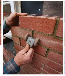
**Let the mortar set.** Once the mortar has dried to a slightly crumbly texture, tool the joints to a consistent depth and shape. Work the head joints before the bed joints for a clean job.
