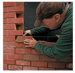
**Slip in the brick.** Hold the weight of the brick in your hand as it's placed. Finish by tapping the end of the brick with the end of the trowel to compress the mortar in the head joint.
