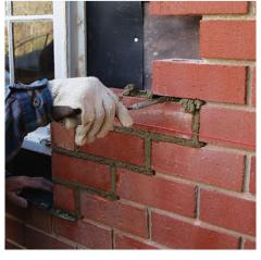
**Pack in mortar.** Fill bed joints between the new brick and the half of the brick above using a  $\frac{1}{4}$ -in. or  $\frac{3}{8}$ -in. tuck pointer. Put a mound of mortar on the brick, and push it in until the joint is packed solid.
