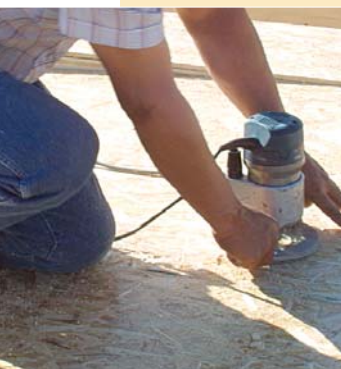
A router removes exterior sheathing at window and door openings. To follow the framing around the opening, you need a plunge-cutting straight bit with a bearing beneath the cutter.
