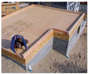
**Plates on deck.** When wall positions are laid out, cut all the top and bottom plates (the long horizontal members) for the exterior walls, and place them on their layout lines.
