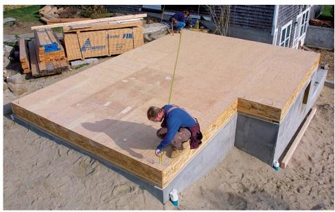
**Equal diagonal measurements mean a square layout.** After snapping chalklines for the longest parallel walls, the author takes corner-to-corner measurements to make sure the corners are square for a perfect rectangle.
