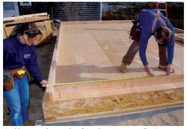
**Stud layout is always taken from the same two walls.** One crew member holds the tape at wall offset while the other marks the stud position (photo above). Even when there is a break in the wall, the layout is pulled from the same place to keep all the framing aligned (photo right).
