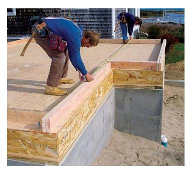
bers) for the exterior walls (top photo above). In this step of layout, we set the plates side by side on the layout line, and every wall-framing member is located and labeled. With this information, we assemble the walls on the floor, then raise them into place. I often call out measurements and have someone cut and hand up the material to keep mud, snow and sawdust off the floor during this crucial phase.
